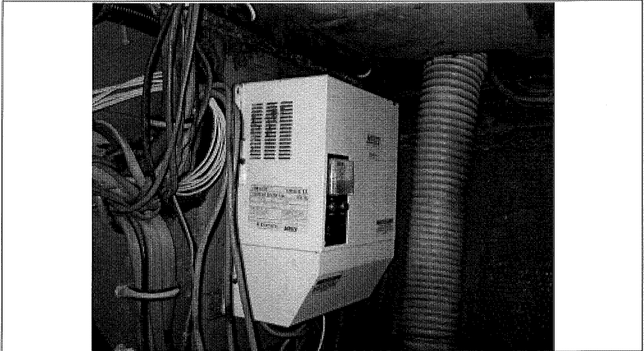
32VDC BATTERY CHARGER
