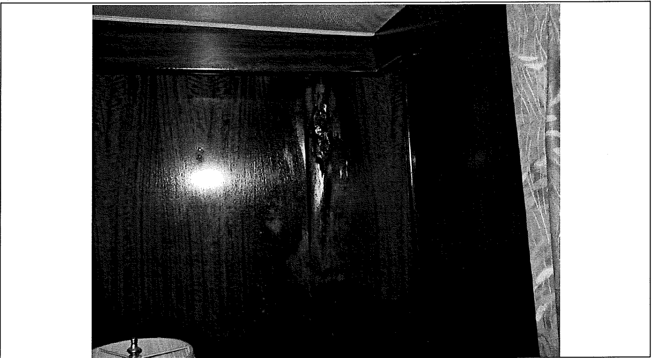
WATER INTRUSION TO AFT STATEROOM
