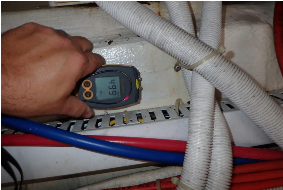
27. Wet moisture readings at inboard transom
