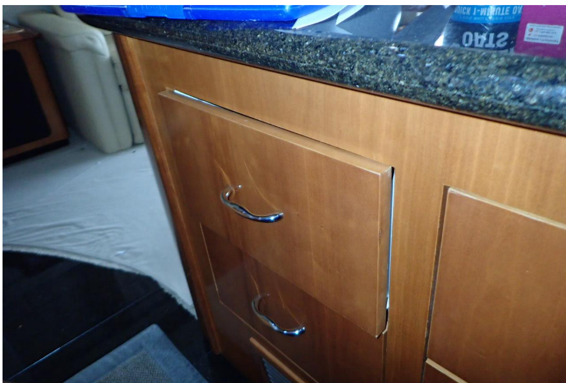
36. Galley drawer does not shut
