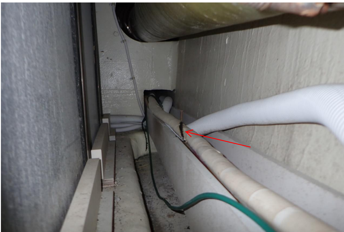
18. Overheating damage
