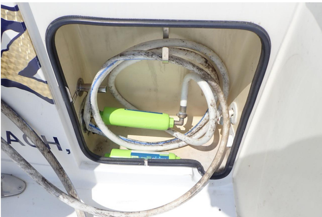
48. Shore water connection
