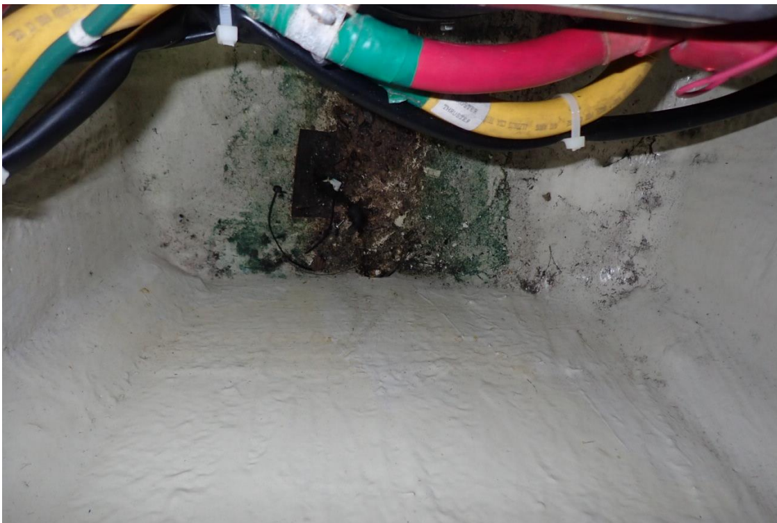
41. Debris in forward bilge
